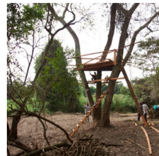
A watch tower is built with the timber from eucalyptus trees.
